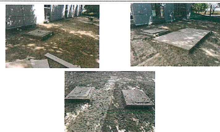
(09) Cisterna Principal, (10) Cisterna Secundaria (Pluvial), (11) Biodigestor
